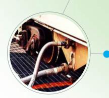
Fibergrate<sup>®</sup> grating and Dynaform<sup>®</sup> structural shapes create slip resistant walkways over existing track pans in refinery fuel car loading zones.
